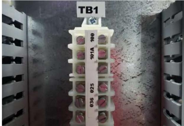
*Figure 2 - Control Wire Terminals*
