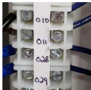
Figure 2 - Typical Control Wire Terminals for a Utility-to-Generator Setup
